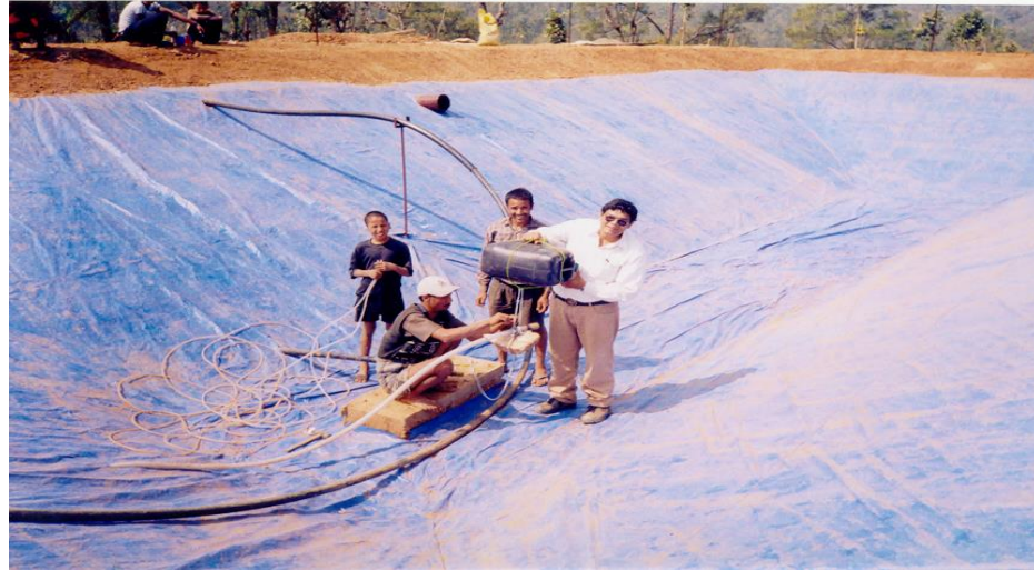
Float being fixed
