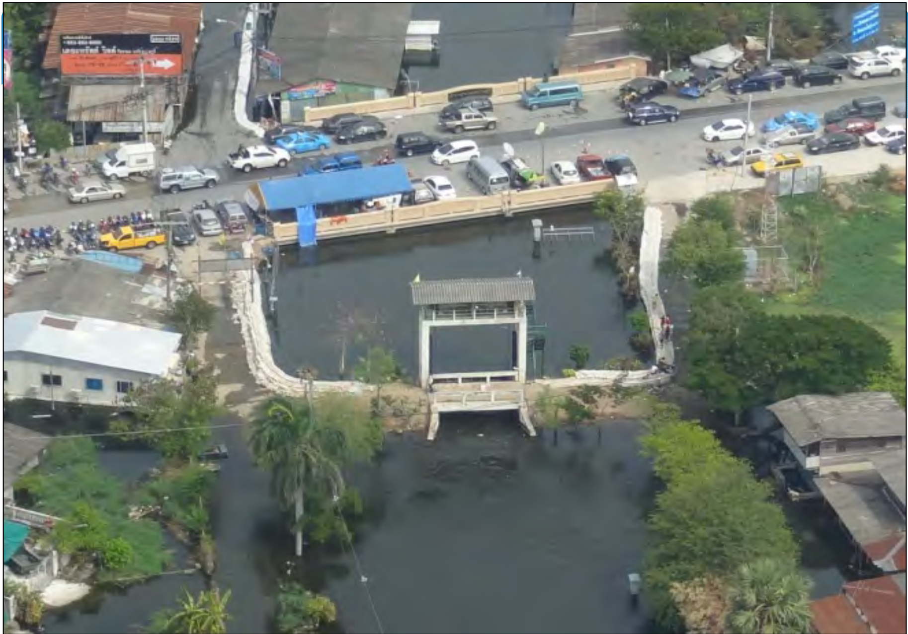
Sluice gate for irrigation not for flood control
