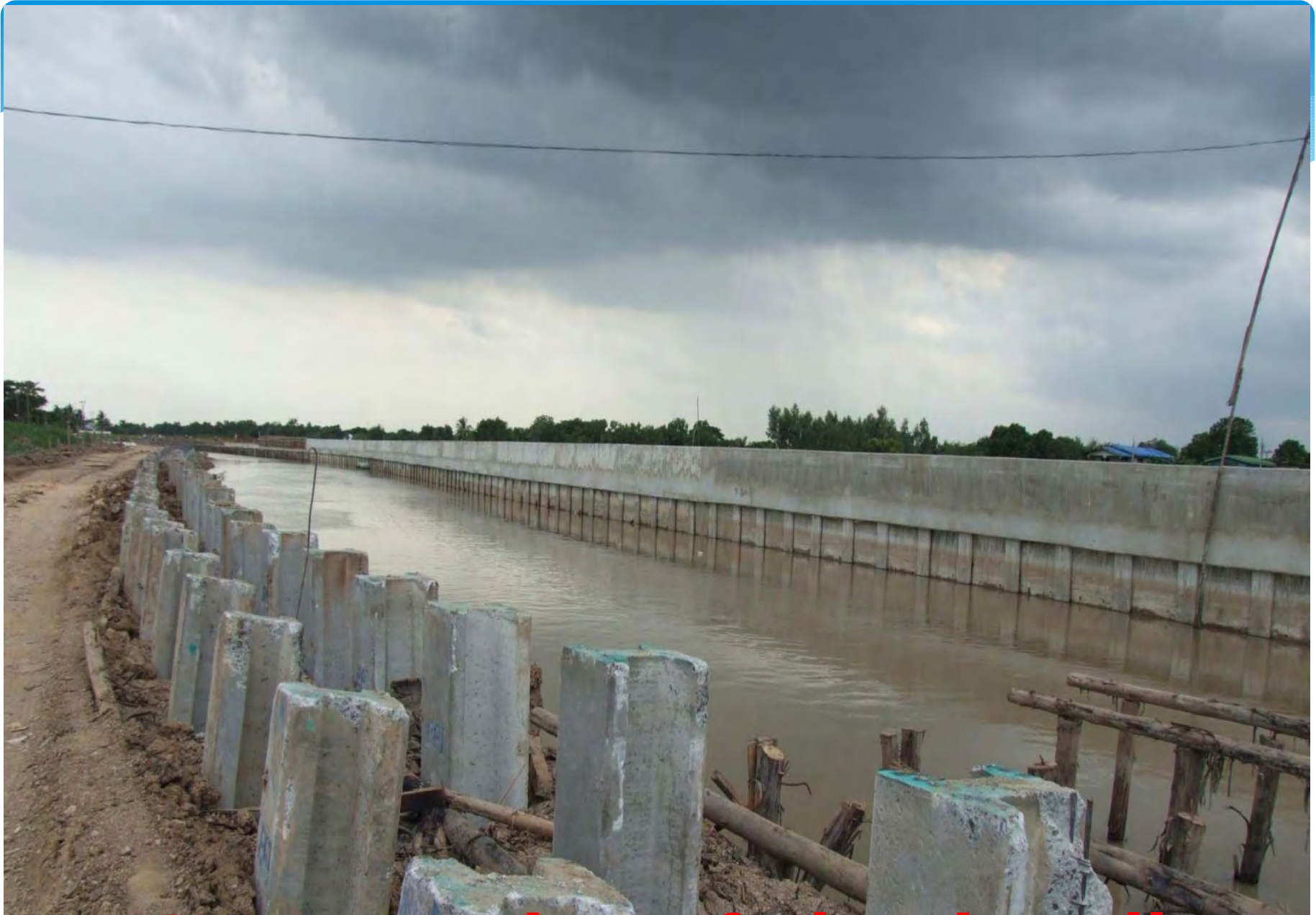
Construction of Flood Wall
