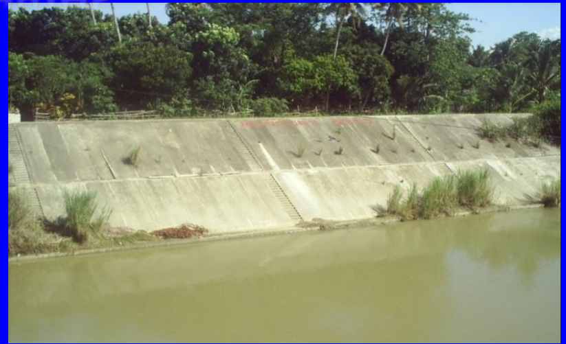
7. Maintenance and additional construction of Mega Dikes.
