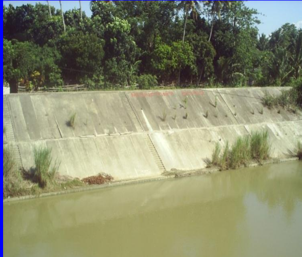
2. Construction of Appropriate/ needed Infrastructure Facilities.
